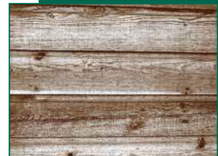
Figure 5-6: Wood siding
