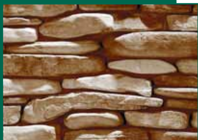
Figure 5-8: Concrete synthetic stone
