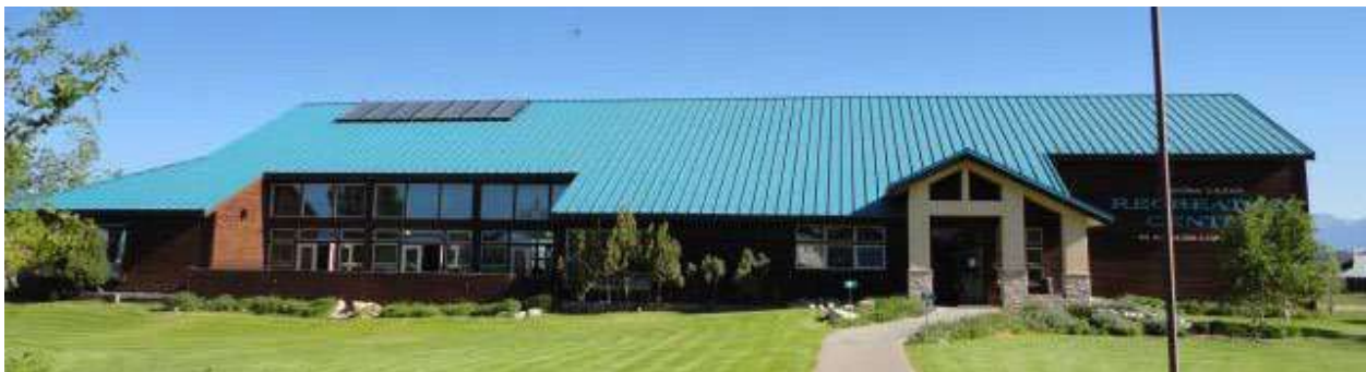
Front facing view from south
